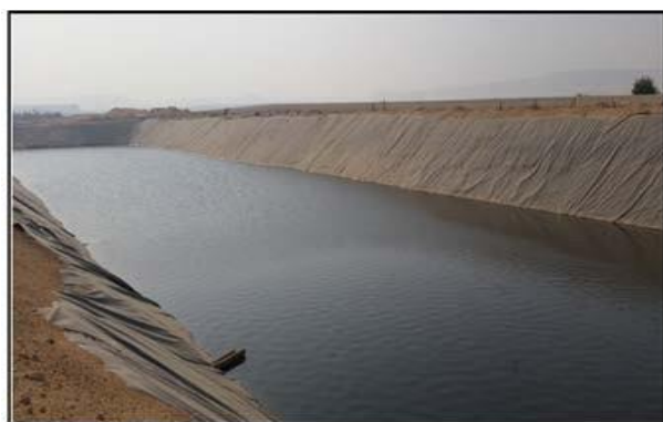
Figure (3): West Assiut combined cycle power plant's evaporation ponds
