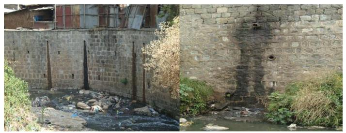
Figure 2. Direct discharge of toilet and domestic sewage to the Shankila River.
