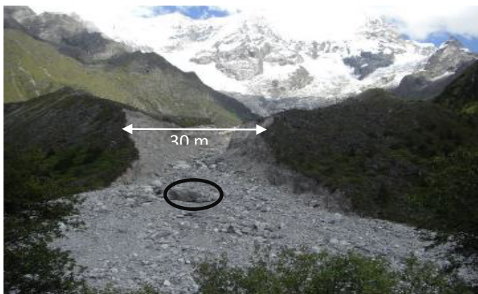
Photo 2. Frontal view of the typical V-shaped channel morphology after the breach. A large dislodged boulder can be seen in front of the breached section.
